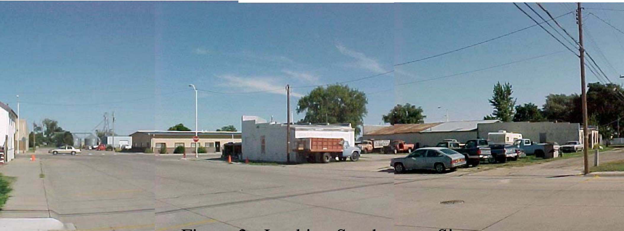
Figure 2 - Looking Southwest at Site
