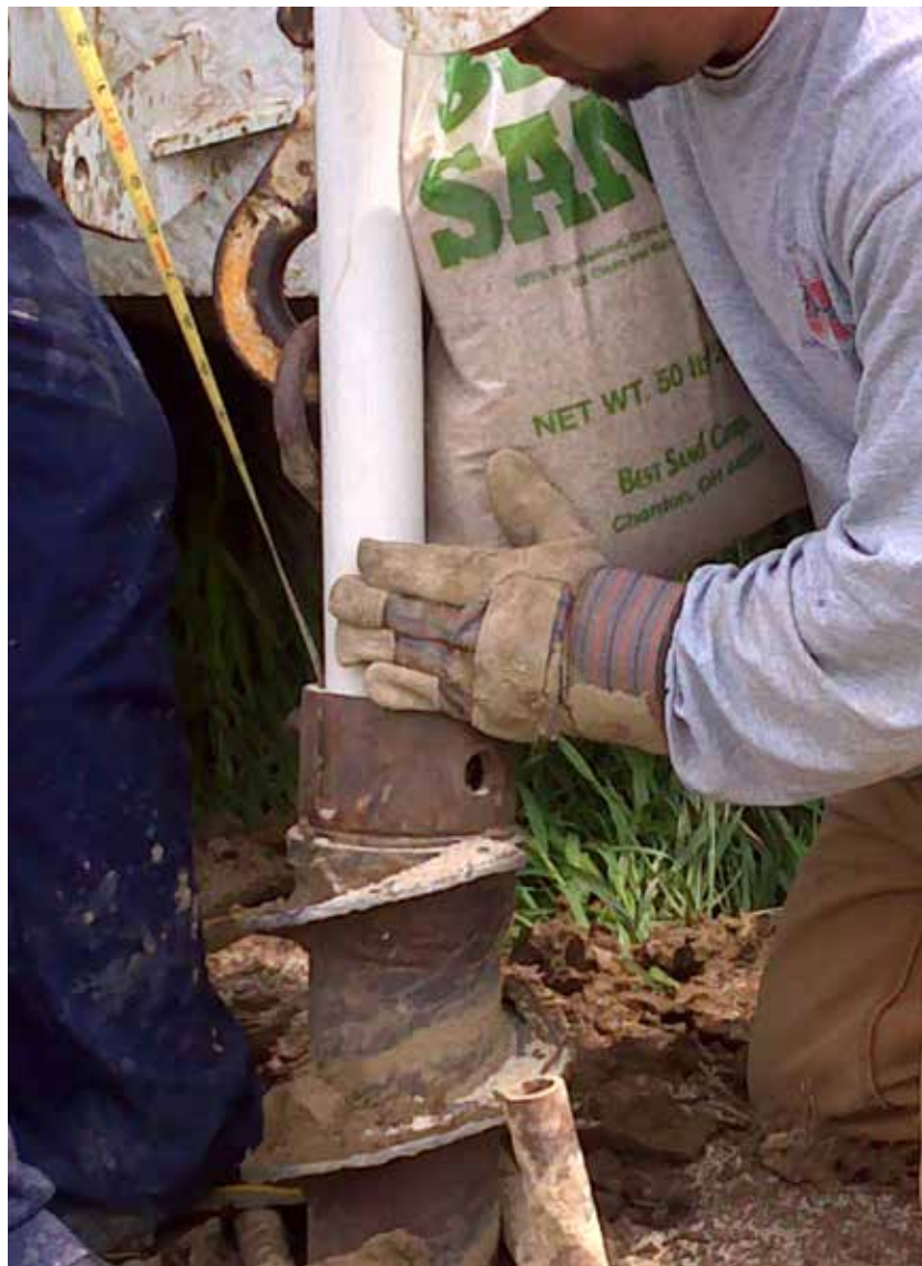
Installing a monitoring well near Clearwater, NE.
